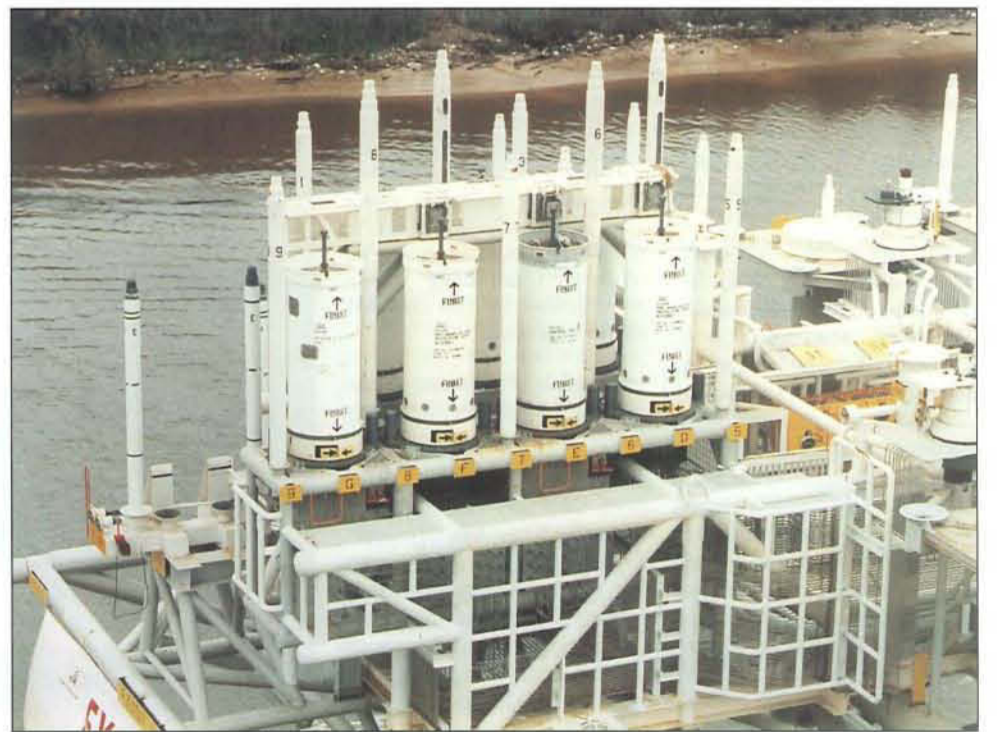
A close-up view of the GEC-Marconi Oil and Gas part of the template.
