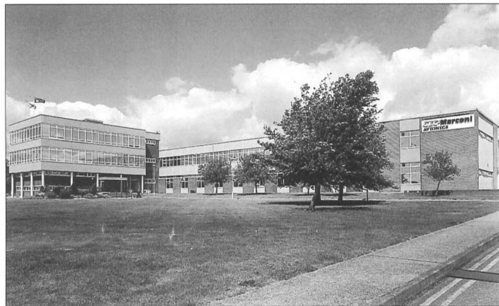
Abbey Works, Titchfield in Hampshire is home to the Power Systems Division of GMAU.
