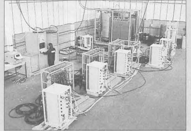
Amerada Hess Hudson Subsea Control System undergoing testing at Nailsea.
