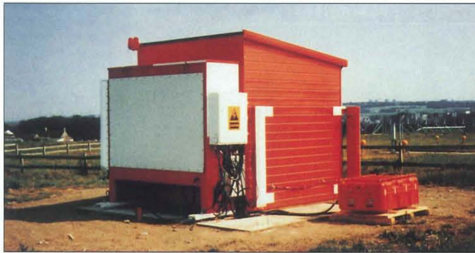
MLS Ground System at Aberdeen Airport.
