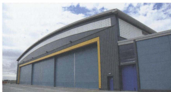
Above: the new BAE Systems Typhoon maintenance facility at RAF Coningsby
