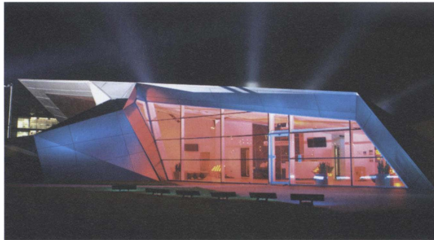
Above: the new face of Samlesbury – the reception building
