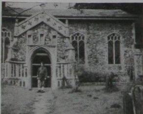
Outside Sweffling church, Suffolk.
