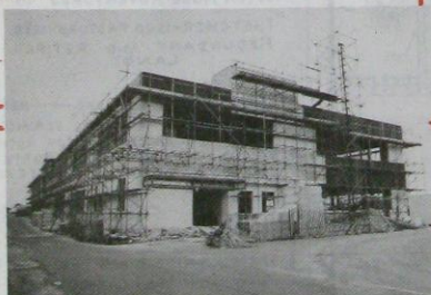
The enclosure of the building almost complete - November 1979.
