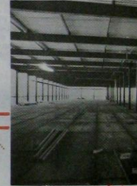
The floor is laid - August 1979.
