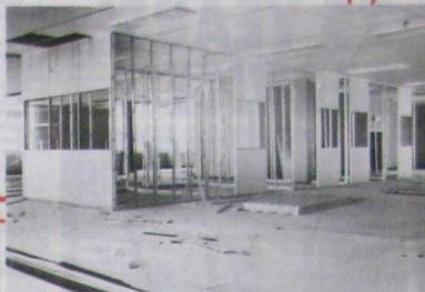
Internal segregation, shows things to come - May 1980
