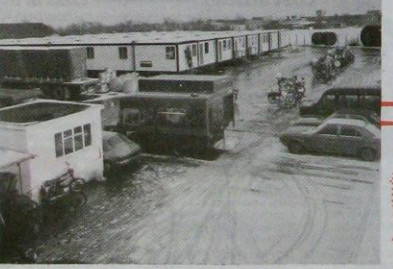
Portakabins take the load while the building grows - January 1979.
