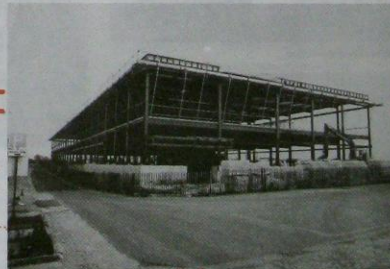
The roof is on! June 1979.
