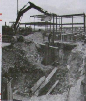
Piles down and steel up - March 1979.
