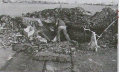
First hole in the car park - November 1978.
