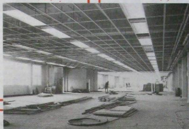
Lighting installed, work can go ahead - March 1980.
