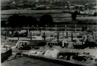
Nailsea premises being developed.
