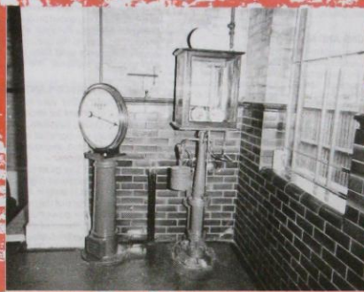
Detail showing brown lining and two gauges
