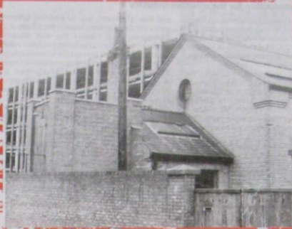
Rear elevation of exterior of building
