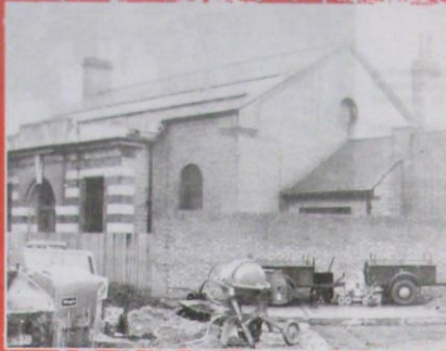
Front elevation of exterior of building
