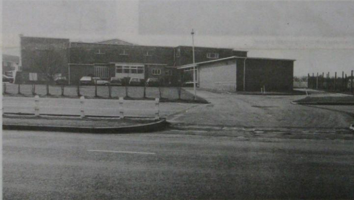
Main entrance to BP (Kent) Club from Bell Lane, Hoo.
