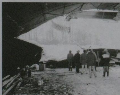
The Blister Hanger – not as designed. 40 ton lift crane at work.
