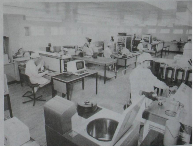
...and after rebuilding This is the Test area fully completed...
