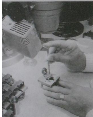
Precision assembly of sub-miniature gyros, which form the heart of Strapdown Navigation systems. The hands belong to Ray Brown who works in the Instrument Technician team in GSD's super clean rooms.
