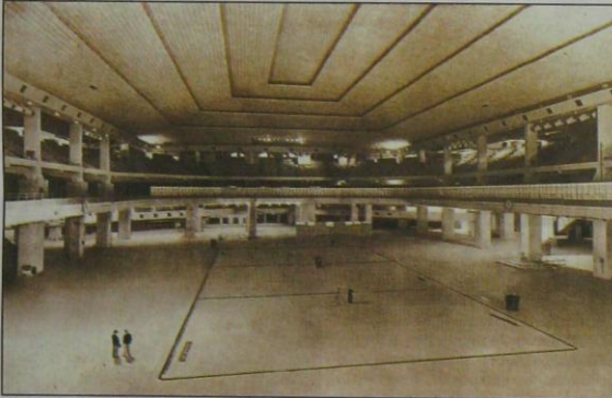
The Central Exhibition Hall of the Earls Court Exhibition Centre, London, showing the adjustable floor of the swimming pool raised to the surrounding floor level.
