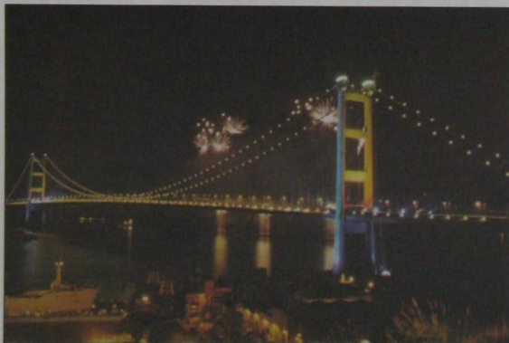
GEC companies have won orders worth more than £175 million for the Hong Kong airport and associated Lantau Link. Featuring a traffic control and surveillance system provided by GEC Hong Kong , the spectacular Tsing Ma Bridge - part of the Link - was opened in May this year. It is the longest suspension bridge in the world to carry both rail and road traffic.
