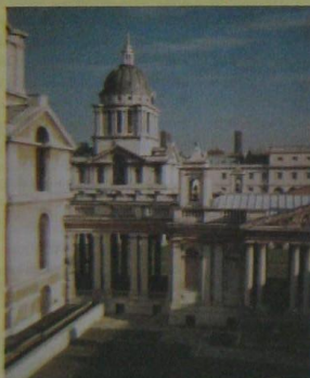
Work will begin on site in April 1998.
