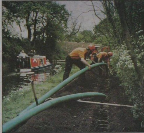
Route canal: Fibreway's nationwide network of fibre-optic cables allows customers to gain access to cable television, data transfer and other high bandwidth applications such as the internet.
