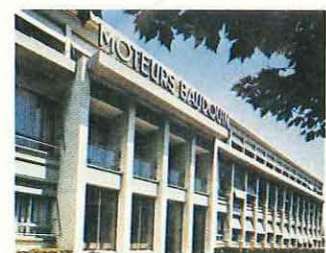
Offices of Moteurs Baudouin S.A., diesel engine manufacturers, in St. Loup, Marseilles. Moteurs Baudouin is a member of GEC Diesels Group.
