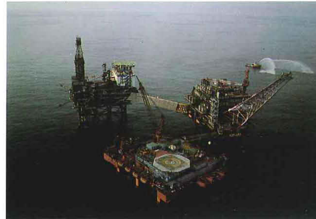
Above and sub-surface stabilisation Photograph courtesy of Total Oil Marine p.l.c.
