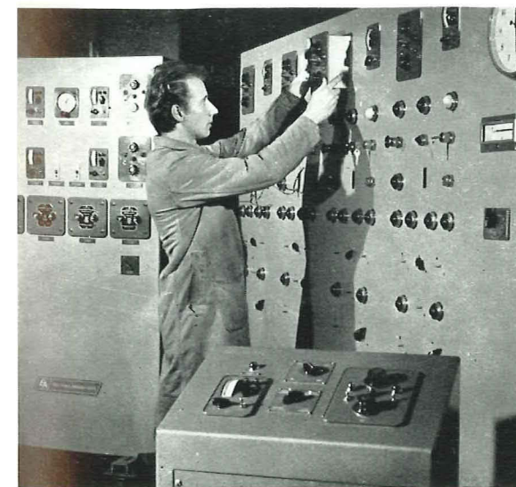
Boiler Control: assembling Elliott "Series 75" automatic control systems for mechanically-fed coal-fired boilers of the type being installed in hospitals, schools and small factories.
