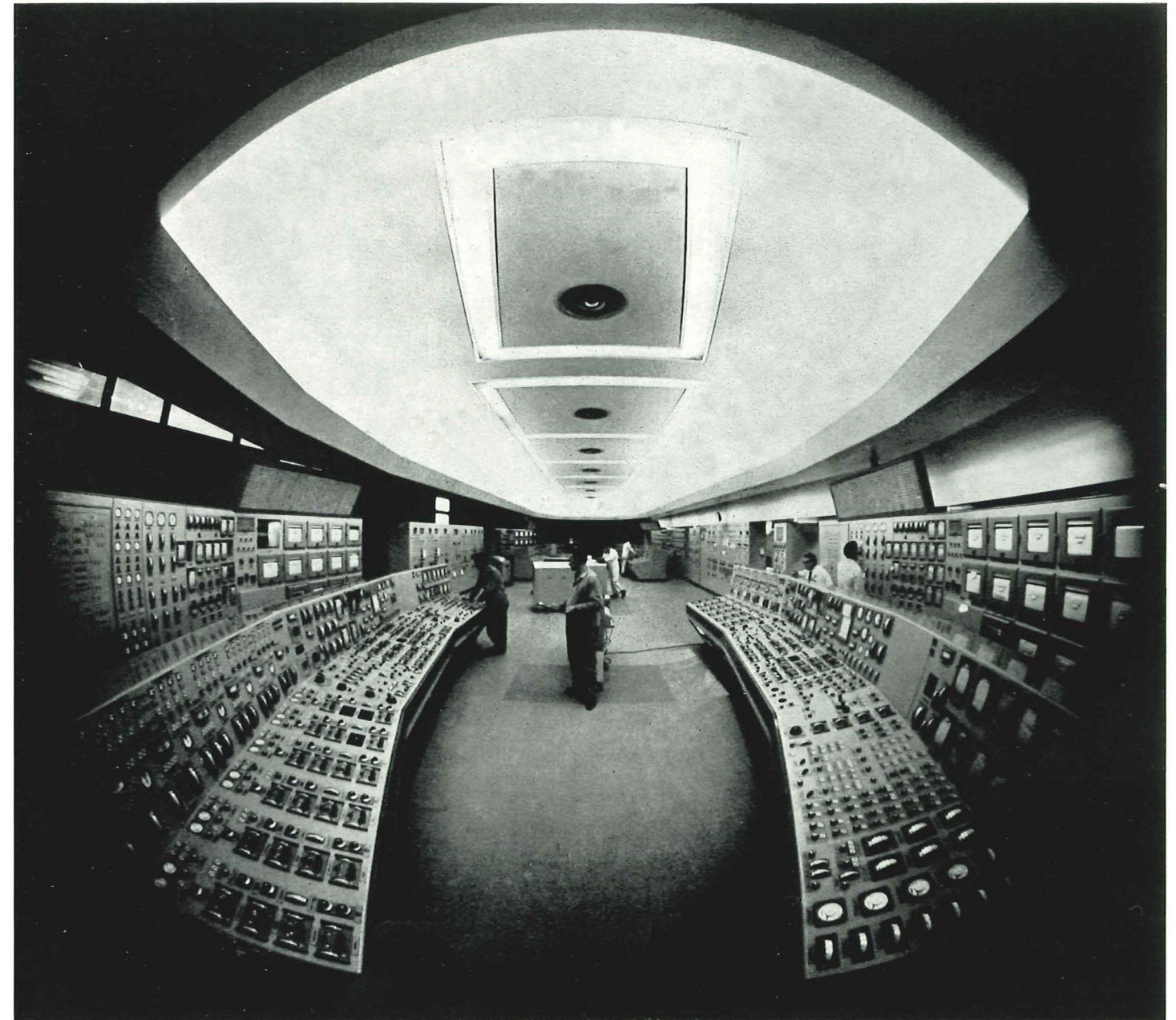
Power Generation: the electronic control room of a 1400-megawatt power station at Tilbury, one of the new stations in Britain for which Elliott-Automation has supplied complete automatic control systems.
