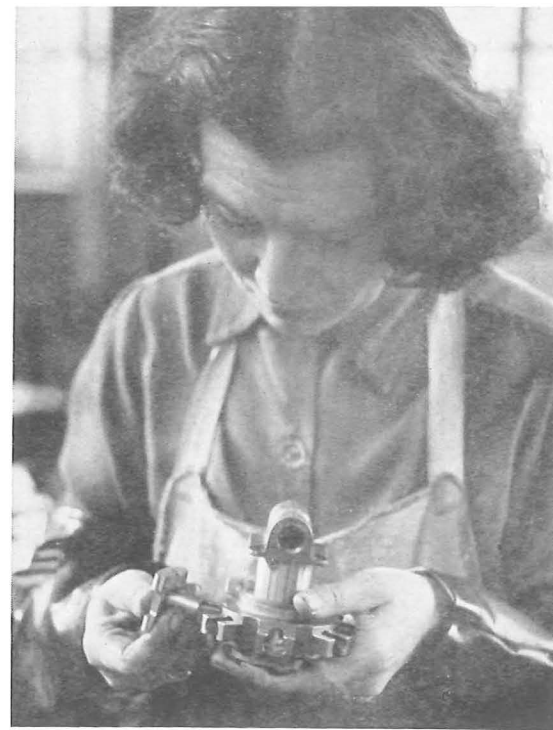
A Sub-assembly. Part of an hydraulic pump.
