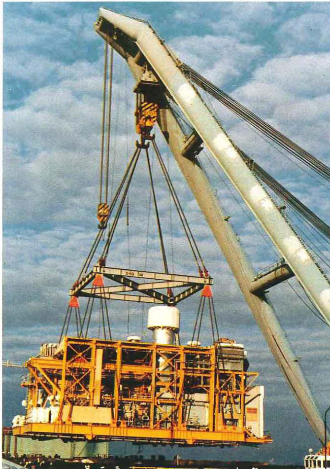
A compressor package for an offshore gas production platform near Bombay. The package, built in Japan, incorporates two 13,300kW gas turbines supplied by GEC Gas Turbines Ltd, Whetstone, Leicester.
