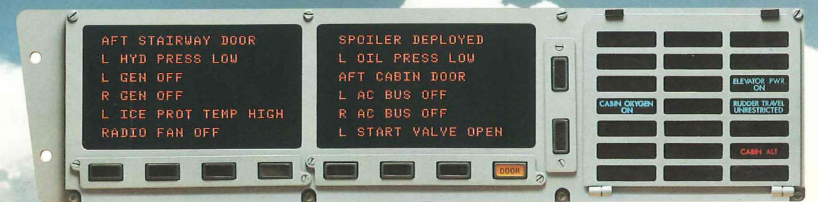
Overhead Annunciator Panel
