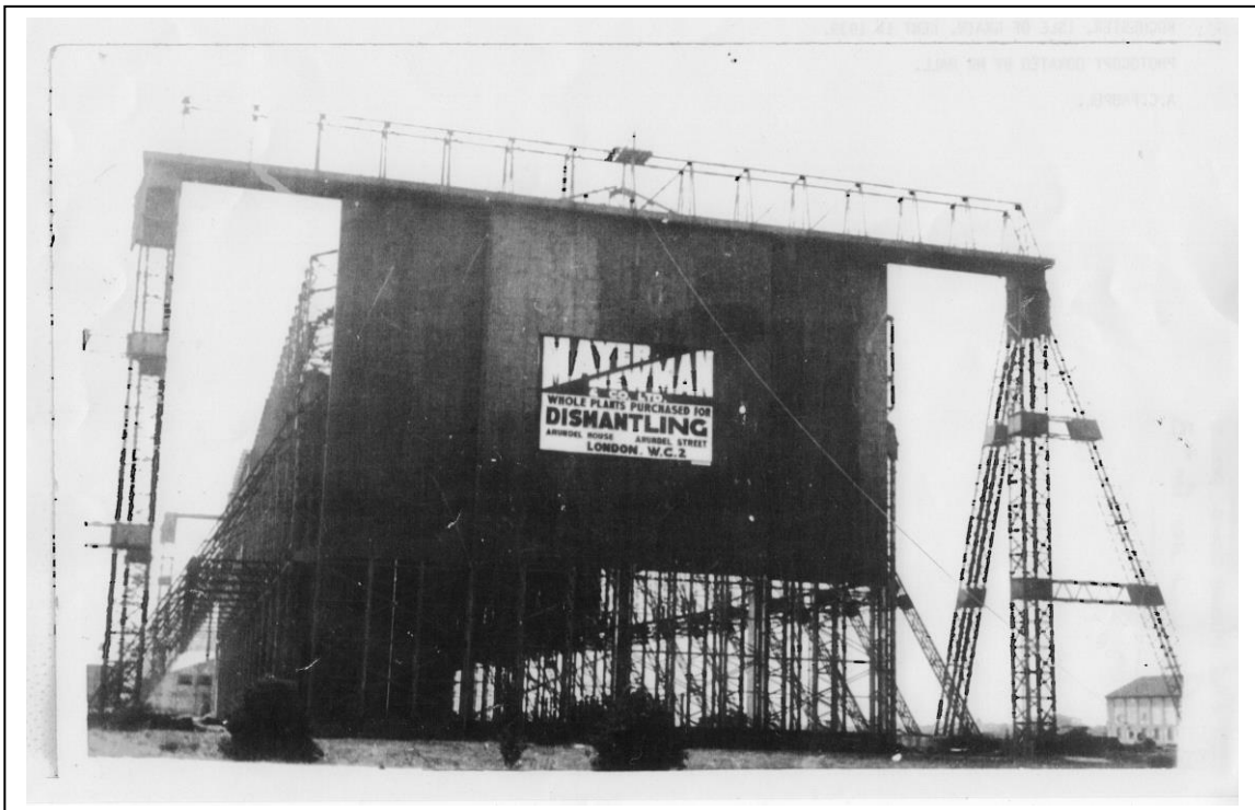
Fig.9. The Steel Hangar at Kingsnorth being dismantled in 1939
