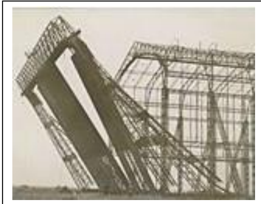
Fig. 10. The Steel shed at Kingsnorth being demolished in 1939
