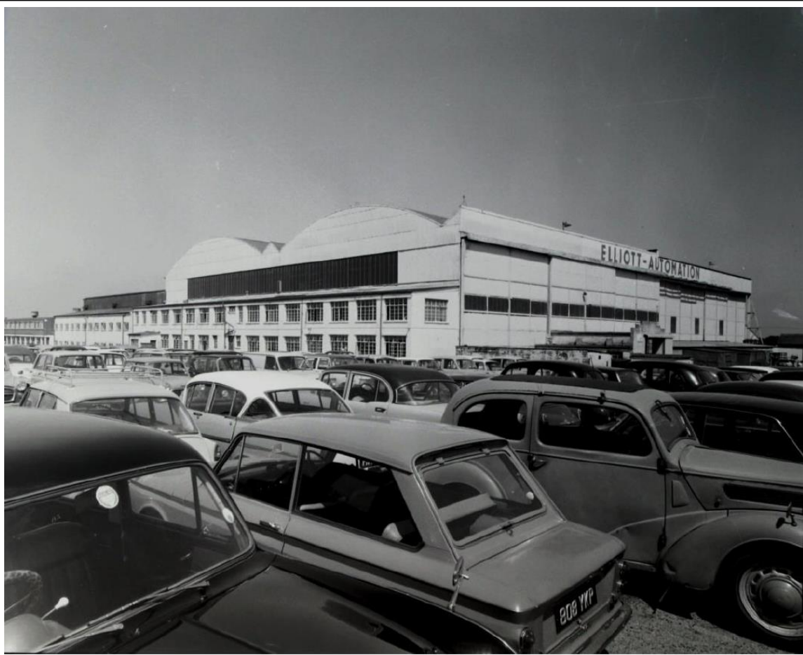
Fig. 5. The Hangars from the South in 1967 showing the round topped pair.
