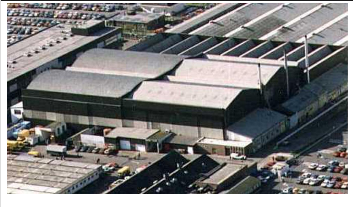
Fig. 6. The Main Site Hangars at Rochester Airport showing the apex roof pair to the North of the round topped pair
