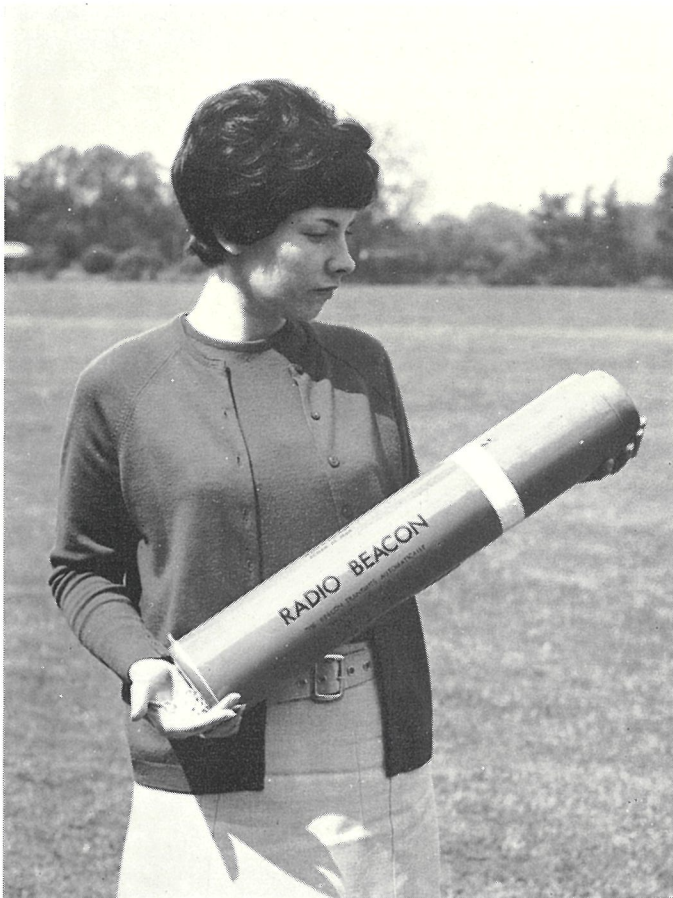
Dual frequency rescue beacon for airliners
