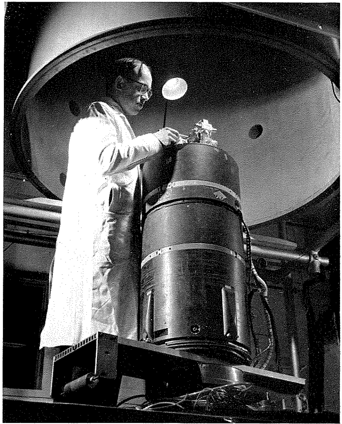
Three-axis attitude control for Skylark sounding rocket
