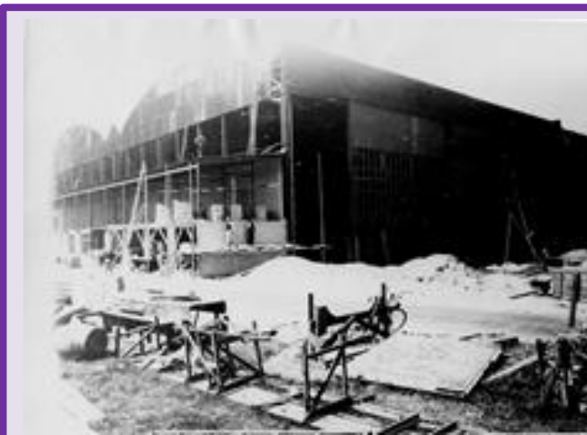
The new Hangars under construction in 1938. (RAA Archives)
