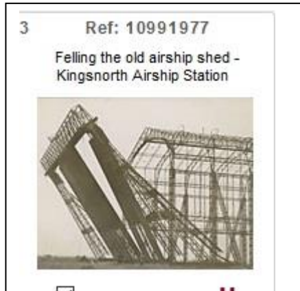
Fig. 10. The Steel shed at Kingsnorth being demolished in 1939
