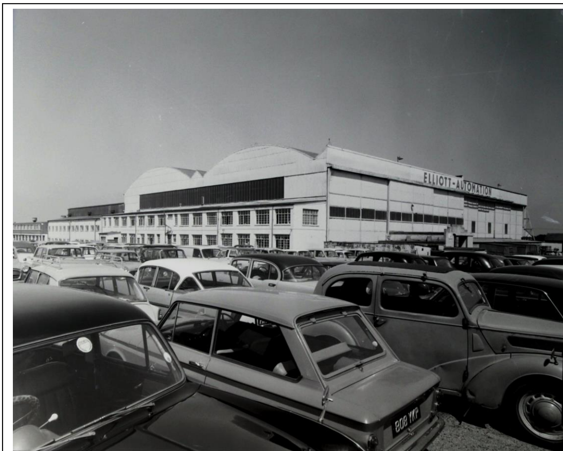
Fig. 5. The Hangers from the South in 1967 showing the round topped pair.
