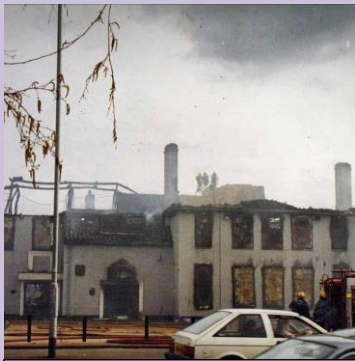
The derelict King Alfred pub after the fire.
