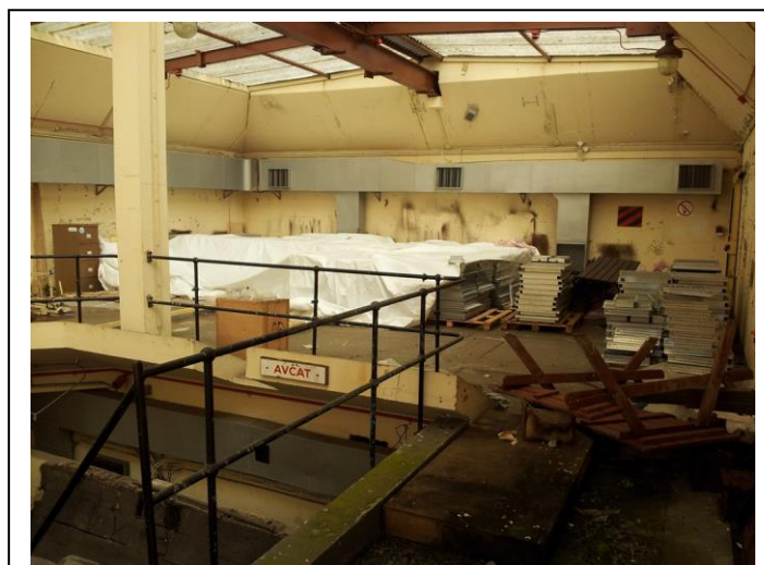
Inside the Test House In 2014
