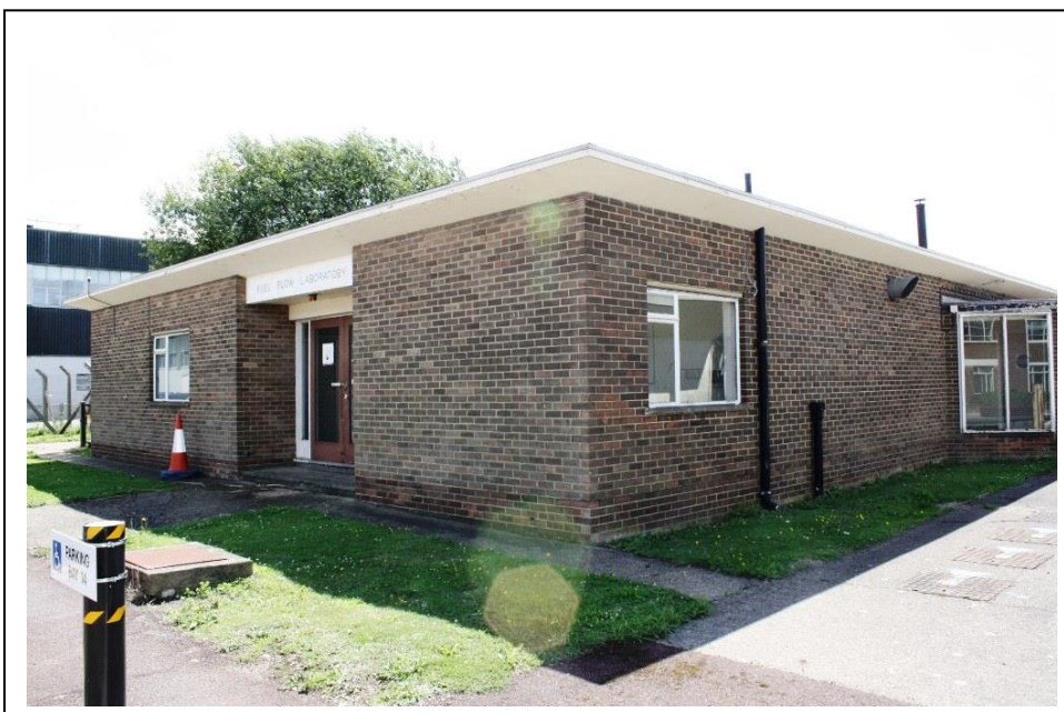
The Fuel Flow Laboratory Control Building today
