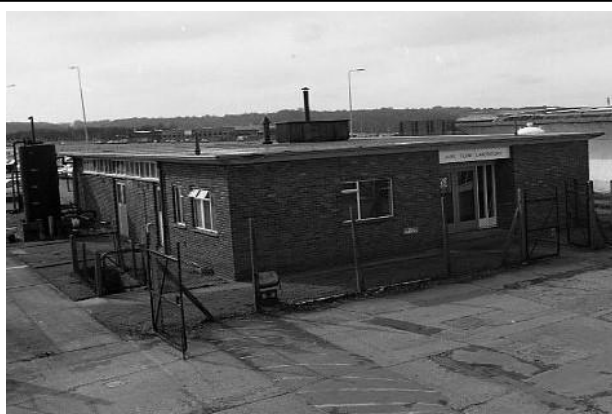
The Control Building about 1964
