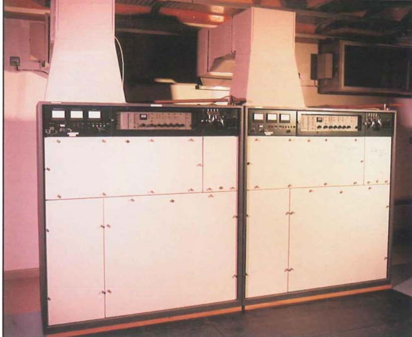
10 kW HF Transmitters
