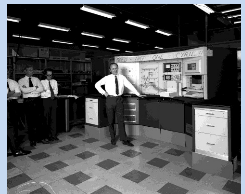
Another of the Leonard Hill pictures showing Cyril Smith of Automatic Test Equipment Division with a Compact ATE for the Clansman a Combat Net Radio system used by the UK Army from 1976 to 2010.
