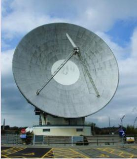
Its first dish, Antenna One (dubbed "Arthur"), was built in 1962 to link with Telstar. It was the first open parabolic design and is 25.9 metres (85 feet) in diameter and weighs 1,118 tonnes.
