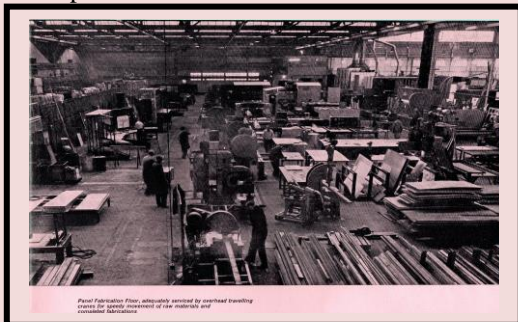
Panel Fabrication Floor, assembly assisted by overhead travelling crane for ready movement of the materials and completed fabrications
