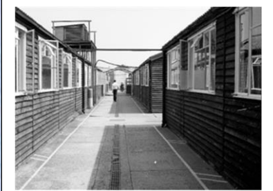
Looking West between Huts 10 and 11
