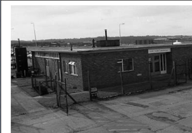
The Control Building
