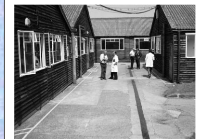
Looking South towards Hut 11
