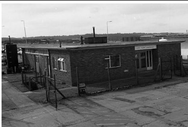
The Control Building about 1964
