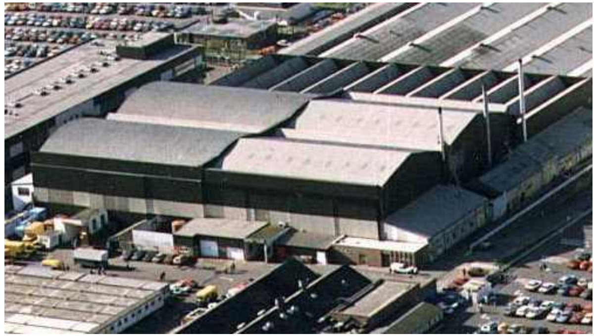
Fig. 6. The Main Site Hangers at Rochester Airport showing the apex roof pair to the North of the round topped pair
