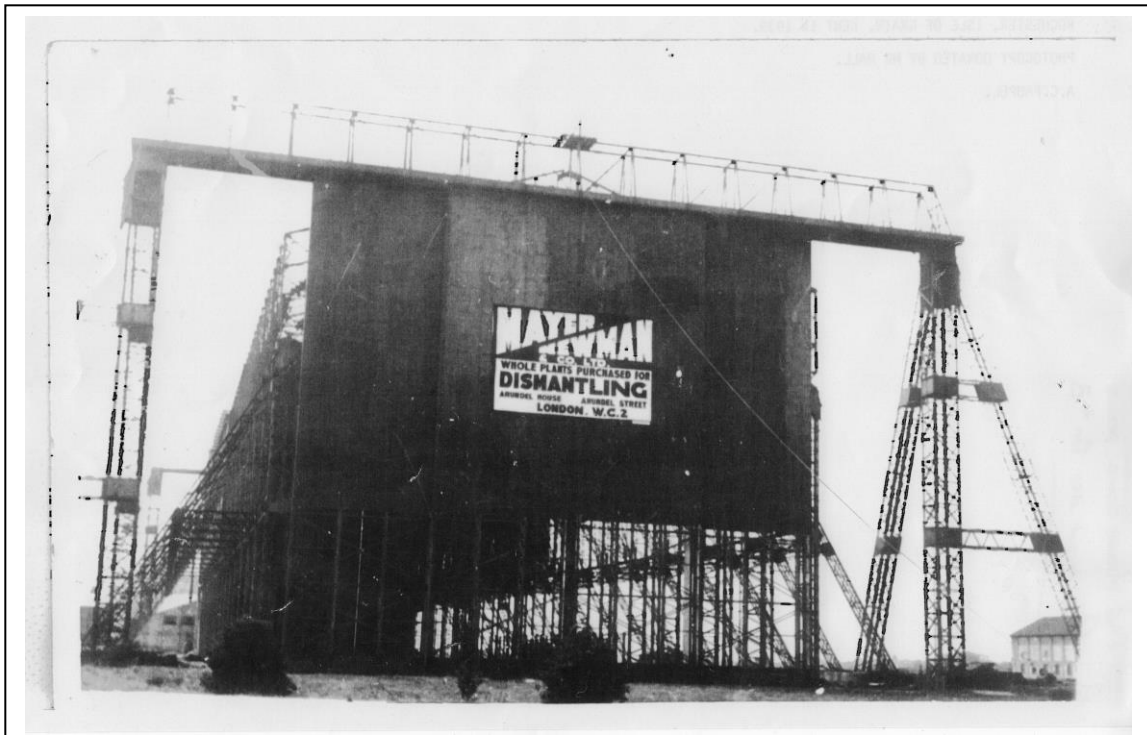
Fig.9. The Steel Hanger at Kingsnorth being dismantled in 1939
