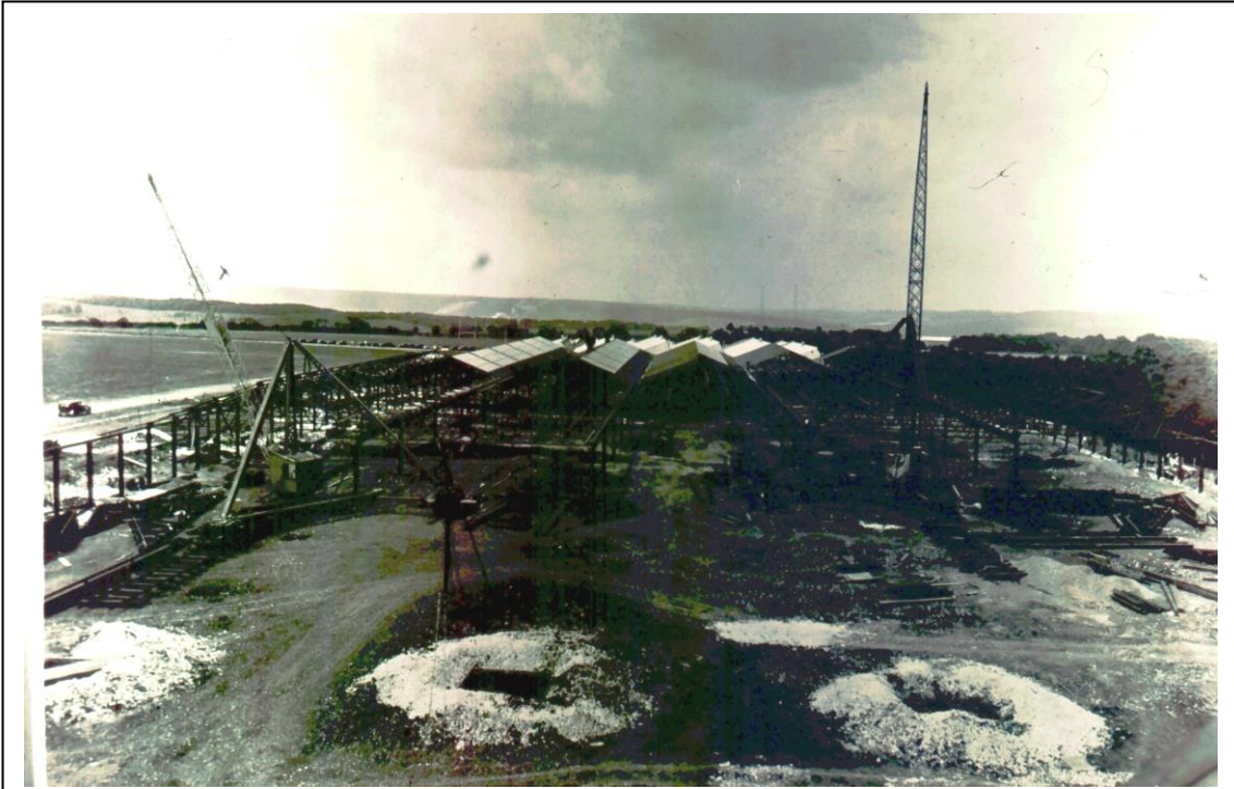
Fig. 2. This picture is looking East in 1938 showing the extensions being built for construction of Stirling Bombers and in the foreground the foundations for the 25' Hanger.
