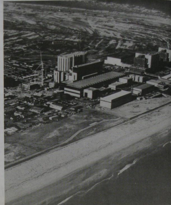
In this aerial photograph of Dungeness, taken for NPC earlier this year, the shape of the point can clearly be seen. Note the two lighthouses, the latest one being situated to the right of the picture. Successive shore lines can also be seen in the form of lines of vegetation formed between ridged peaks of shingle created by powerful tides moving the shingle over land. As a matter of interest Advanced Gas-cooled and to the right is the
