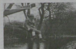
Swinging derrick - commissioning.
