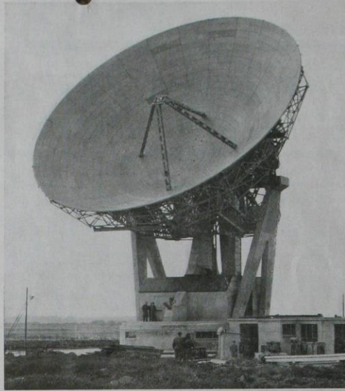
The giant aerial at Goonhilly Downs in Cornwall, which is being used to track the 'Telstar' communications satellite, is steered by instructions from a National-Elliott 803 Computer. (Photograph by courtesy of H.M. Postmaster General)
