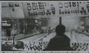
Pictured is the rod winding into coils prior to the finishing end.
