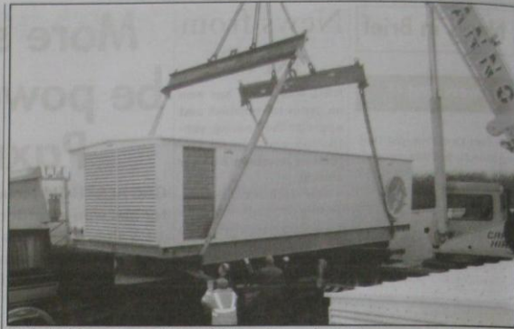
Woods of Colchester's Airpac Division is helping staff at one of Britain's major supermarket companies keep cool.
