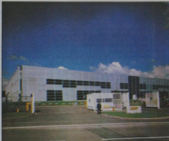
GPS CMOS (complementary metal oxide semiconductor) facility at Plymouth, UK.
