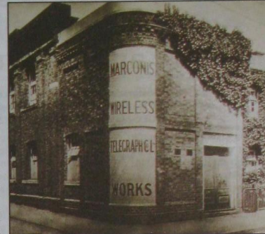
The Marconi factory at Hall Street, Chelmsford. This was the first wireless factory in the world - 1899.
