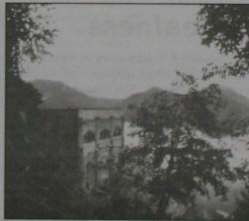
View of Alouette Lake hydro station today, from above the penstock.
