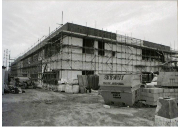
The Phase III Building under construction around 1980
