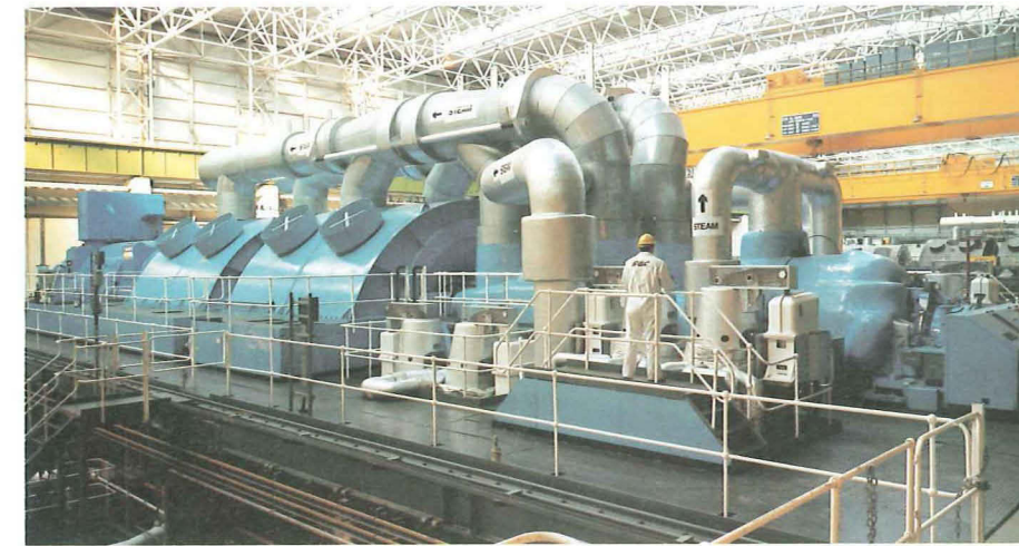
The first 660MW turbine generator installed in the Torness power station in Scotland. It began to generate electricity this year.
