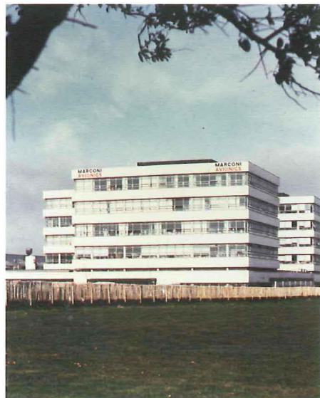
Towers Site, Airport Works, Rochester
