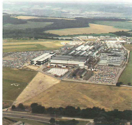
Aerial view of Airport Works, Rochester
