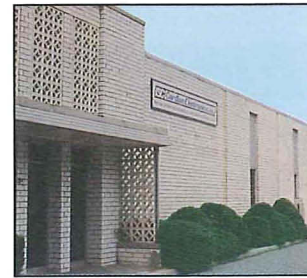
Woodbury, New York ISC Cardion Electronics, a US-based defense electronics company, is a worldwide manufacturer of radar, nav aids, display and communications equipment for civil and military customers. Its facilities are in Woodbury and Holtsville, New York.
