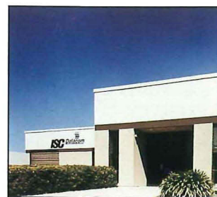
Sunnyvale, California ISC Datacom designs, develops and manufactures RF modems and RF data link communications products.
